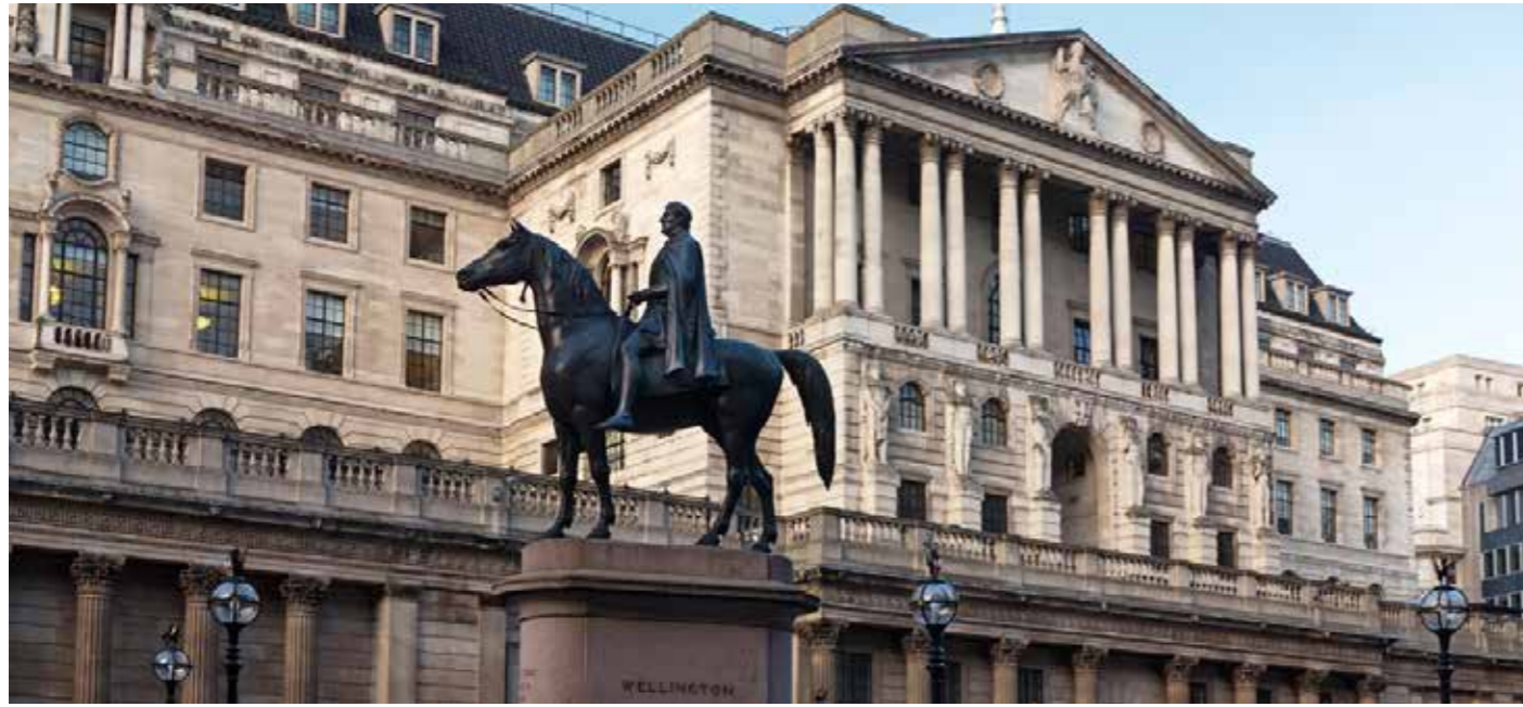
The Bank of England's iconic headquarters in London, heads up regional branches forming a UK network
