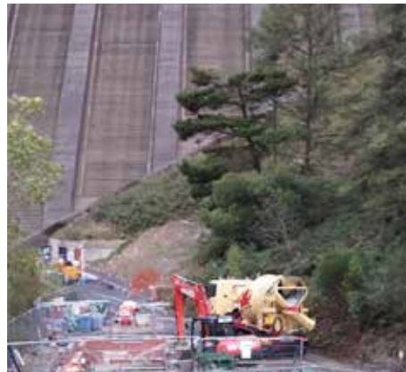
Work takes place in the shadow of the dam
