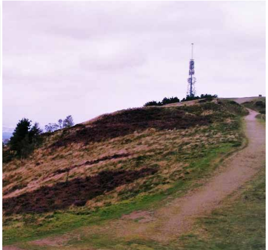
Improve your connection – Unitron, a Telford-based company and business partner of Connexis, provides high speed wireless internet access via the mast on top of the Wrekin
