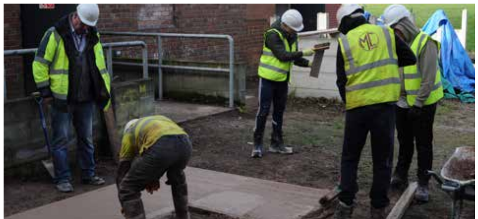
Paving demonstrations taking place at Telford College's construction centre
