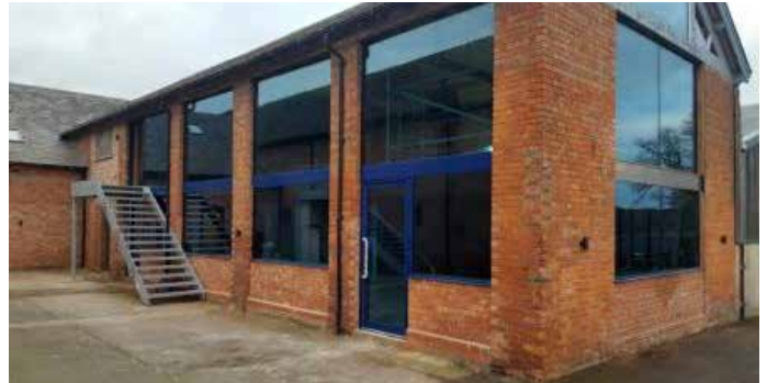
Fresh look - the latest brick pillar barn includes large glass sheets
