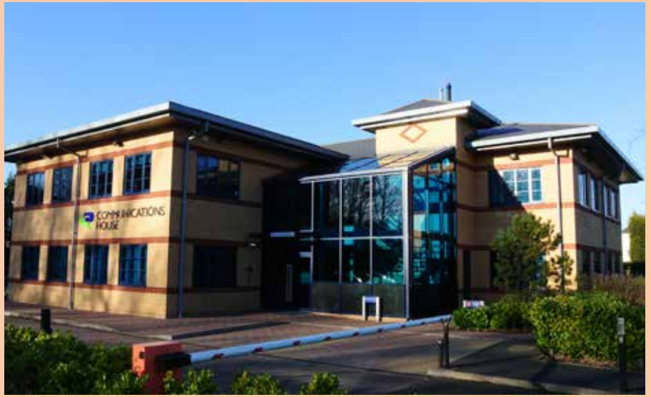
Communication House, Network Telecom's headquarters at Hadley Park in Telford
