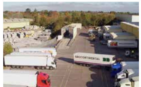
Grocontinental's purpose-built 35-acre complex, providing a base for its cold storage and logistics services
