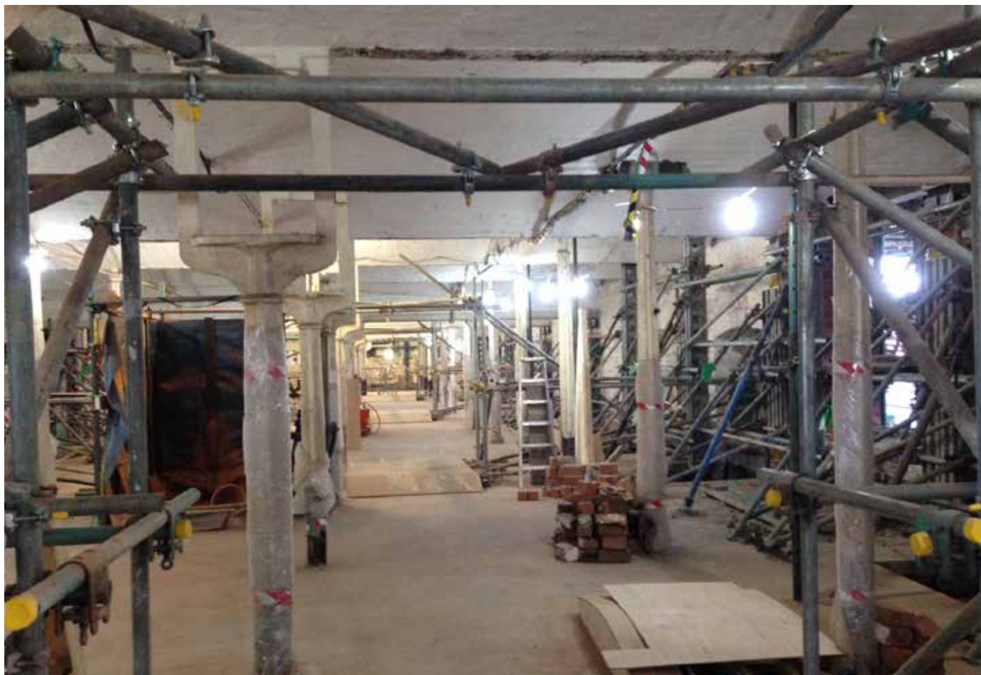
Miles of scaffolding is propping up external walls internal walls, window frames, doorways, floorboards, stairways and lots more besides
