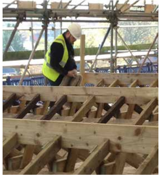
A workman carries out remedial work on the roof of the historically important Ditherington structure
