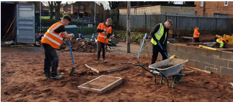
The construction and groundworks training area at Telford College
