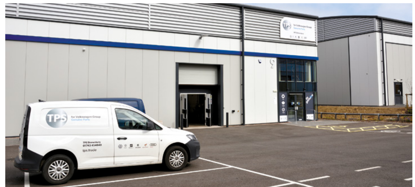
TPS at Unit 9
