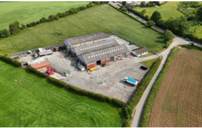
Thorne Works at Dorington
