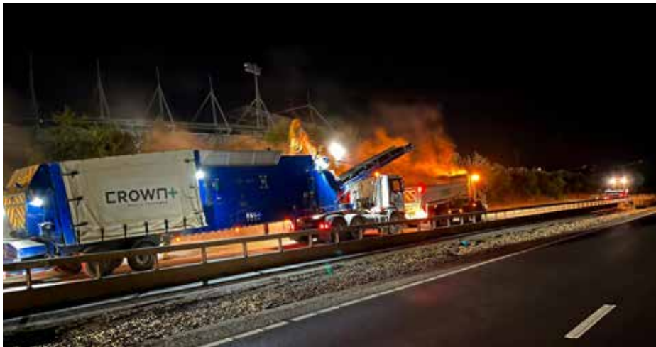
Night repairs by the Crown Plus team
