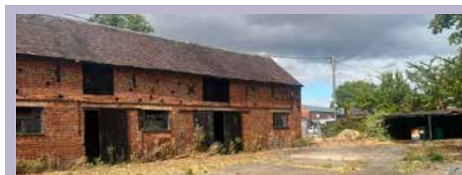
One of the two buildings set to be renovated
