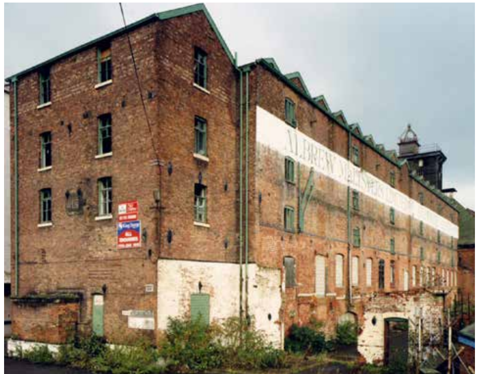
Ditherington Flax Mill has long been the subject of development negotiations
